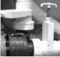
3. Be sure all pump and heater unions are secure. Each pump has 2 unions and the heater has 2 unions. A newly delivered spa may have loose unions caused in transporting the spa. Check that all slice valves are open, in the up position. The slice valves may become closed during transportation of the spa.
