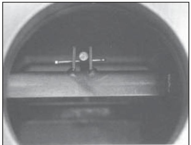
16. Next working through the flue hole behind furnace, line up rod between the two posts on the sliding smoke damper. Then line up the three (3) holes for cotter pin insertion, this procedure will test your patience. It's helpful to have a flashlight and another person positioning the rod.
