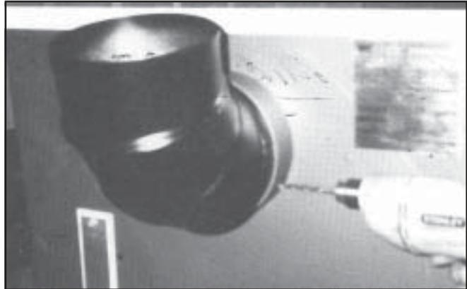
19. Attach flue pipe to flue collar. Flue pipe (6") fits inside
