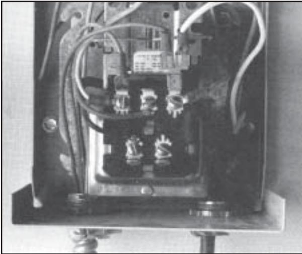
6. Attach low voltage thermostat No. 18 up to 30 ft. run No. 16 to 15ft. Run (purchase locally) to terminal plate, screws identified with letters G & R. (Generally top row center, bottom row right). Snake wire through holes in top of box. Replace outer covers & control knob. Under no circumstances should you attempt to plug in main power cord until all wiring and covers are in place. NOTE: A ground power cord plug is provided; however, local codes may require fuse box mounting.
